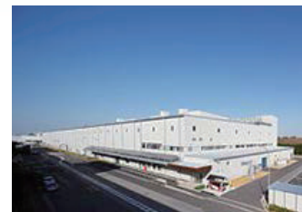
The waterborne paint Plant
