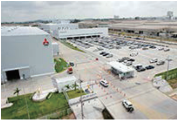
Mitsubishi Motors (Thailand) Co., Ltd. (MMTh)
