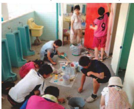
Renovation of elementary school toilets that were struck by the disaster
